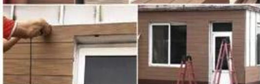
3. Fix the wall cladding
