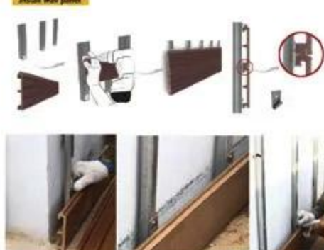
2. Fix the starting clips
